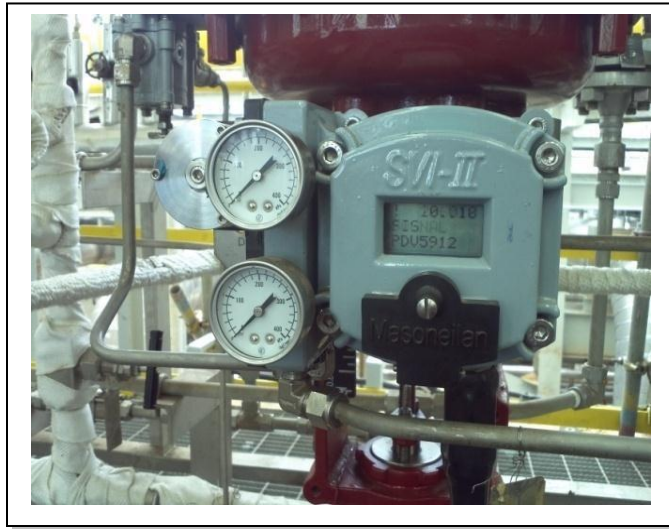
Gambar 2.7 Positioner control valve .
